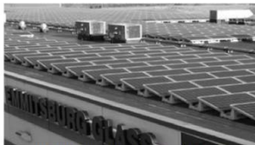
Emmitsburg Glass' solar panels will produce 276,004 kilowatt hours/year, allowing Emmitsburg Glass to go 100% solar.
